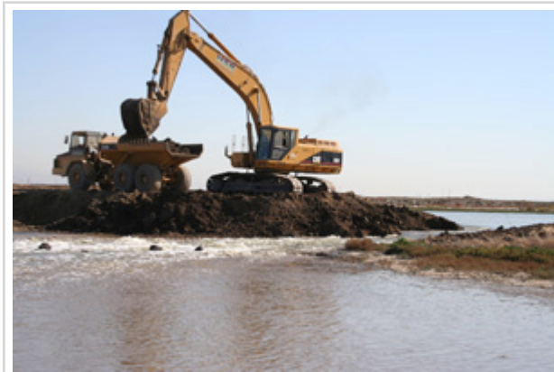
South Bay breaching at Eden landing.
