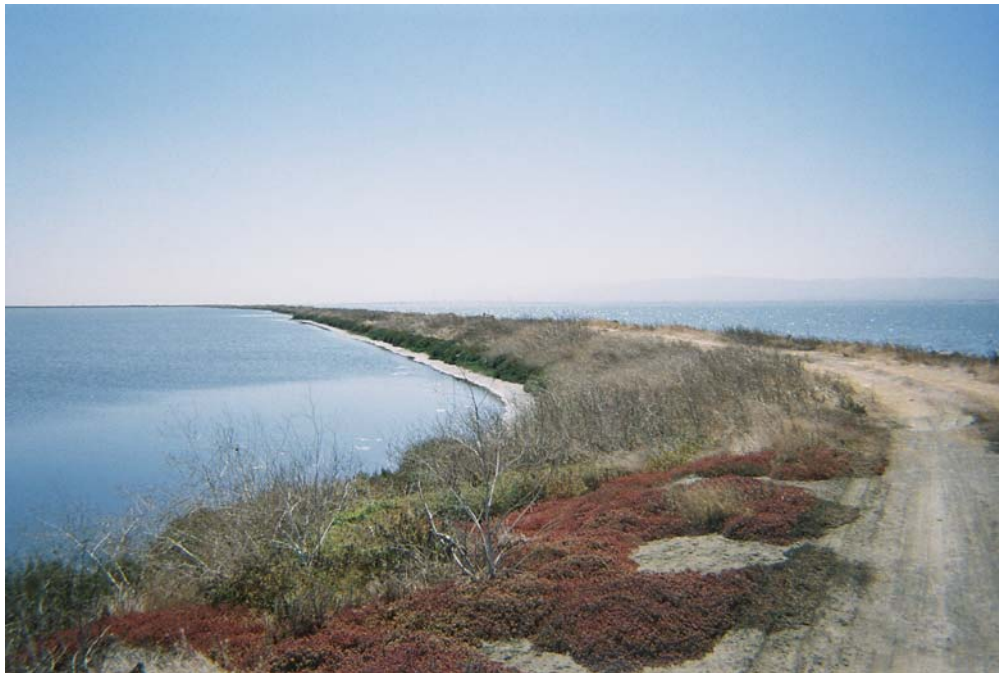
Photograph 2: Example of levee with vegetation slope protection (Pond B2 Northwest)
