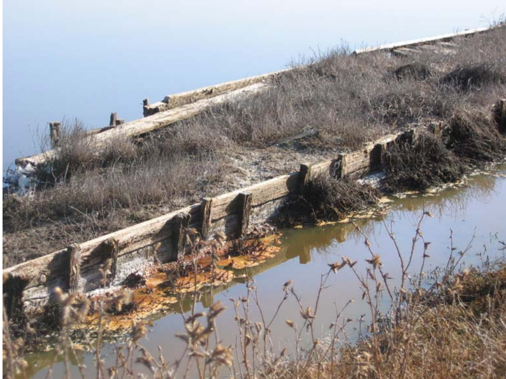
Photograph 5: Example of levee with wood shoring slope protection (Pond B10 North)
