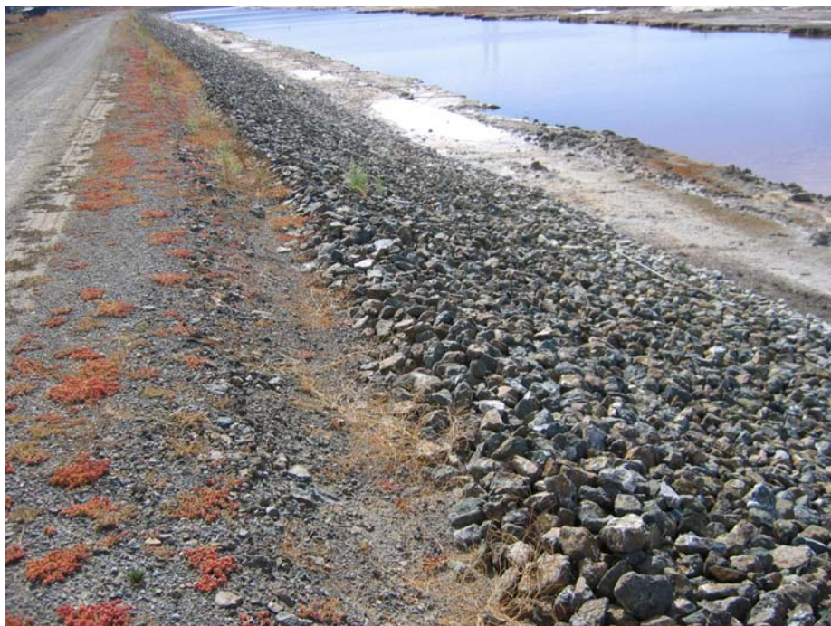
Photograph 4: Example of levee with engineered riprap slope protection (Pond SF2 Southeast)
