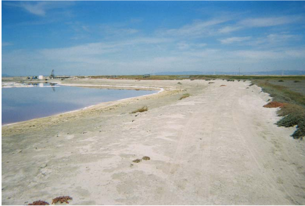
Photograph 1: Example of levee without slope protection (Pond R3 Northeast)
