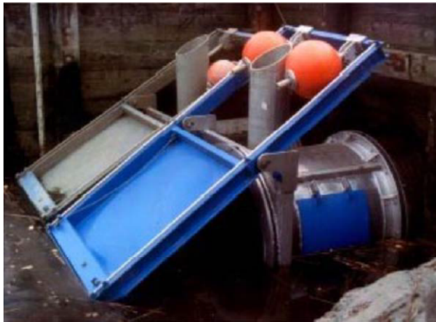
Typical Tide Gate Across Slough
